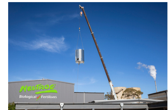
New brewing tanks being lowered into the updated Liquid Room in 2022
