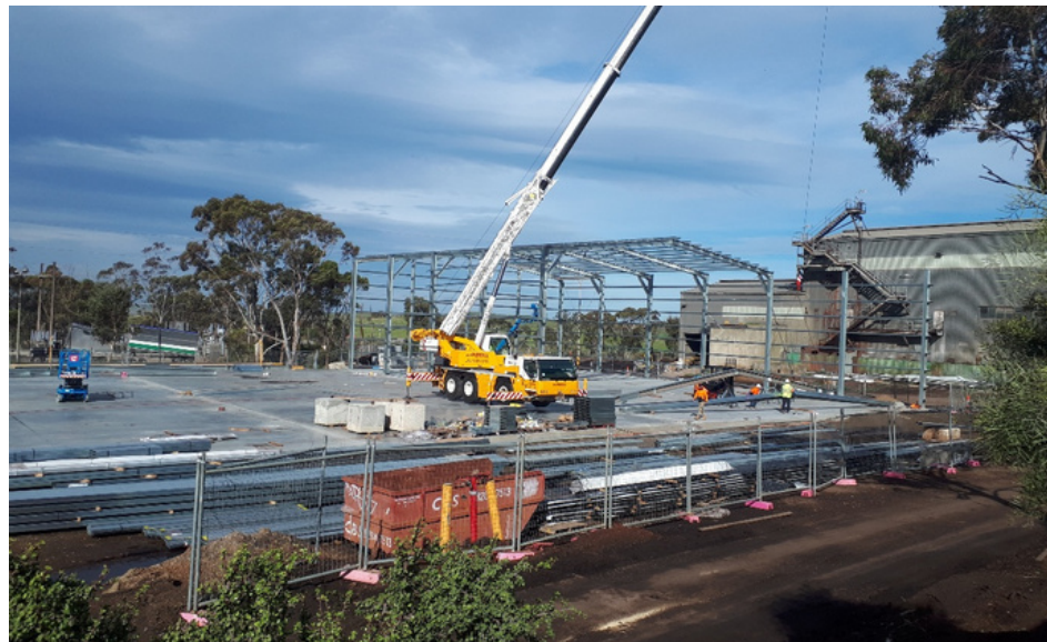
The new 2000m2 warehouse being built in 2019
